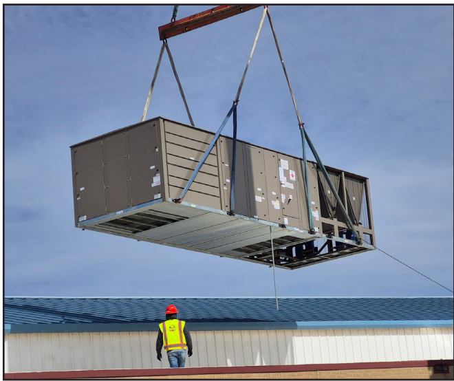
The HVAC workers use a large crane to replace the old rooftop unit at the school. Photo Credit: Eugene Kaiser
